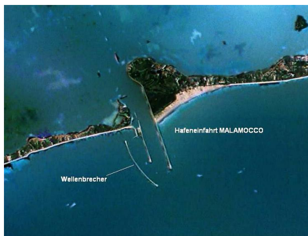
Picture 2: Malamocco harbour entrance with wave breaker
