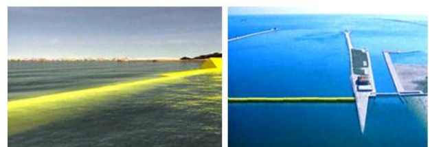
Picture 5: Construction of the protective wall
